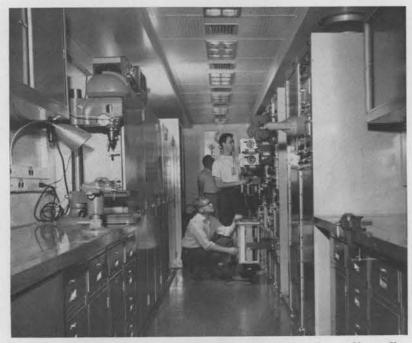
NEW FIELD TEST TRAILER at Livermore Laboratory offers all the comforts of home plus the latest in instrumentation equipment. The 40-foot trailer is equipped with air conditioning, refrigerators, telephones, electric lights, work bench, power tools, radio receivers, and microwave telemetry instrumentation. Checking equipment for use by the Nuclear Support Section (8123-2) are (front to rear) Stewart Ingham, Jim Blanchard, Dick Read, (all of 8123-2).
